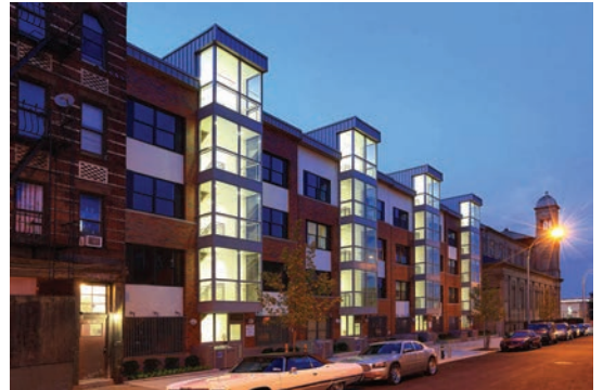
Monsignor Anthony J. Barretta Apartments, East New York, Brooklyn Above right: Exterior Right: Night view—the glazed stairwell acts as a lighthouse on the street
